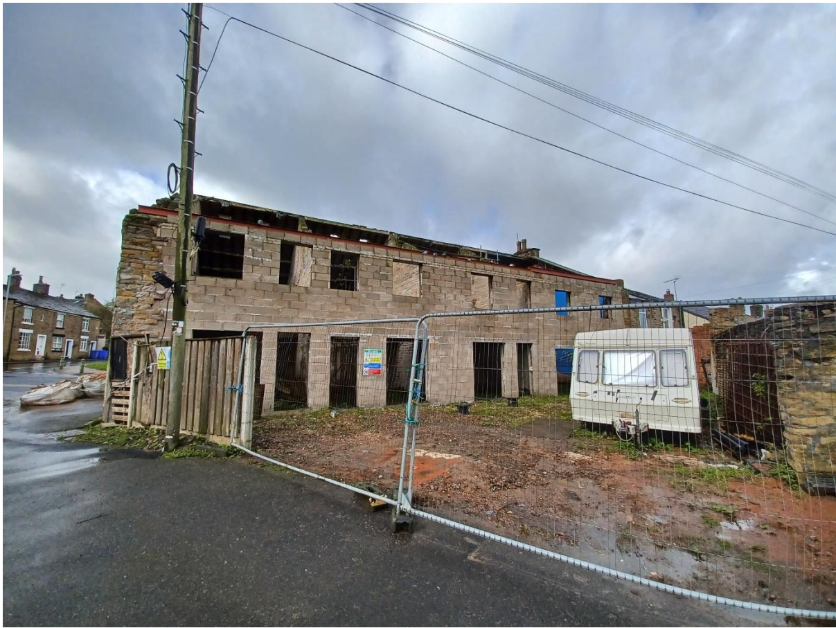
Photo 2: Rear elevation of application building.
